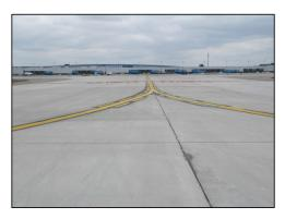
Gives warning that a runway hold short position marking is located ahead. Especially helpful during conditions of reduced visibility. Be prepared to STOP at the runway hold short position until cleared onto or across the runway by ATC.
