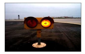
Used to identify the holding position for a runway especially at night and during periods of low visibility. Elevated runway guard lights are amber.
