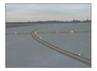
In-pavement runway guard lights are co-located with runway hold bars, above-ground runway guard lights, and hold position signs. These lights are yellow.
