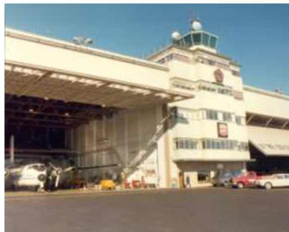
Photograph 2: Willow Run Airport Hangar 1
